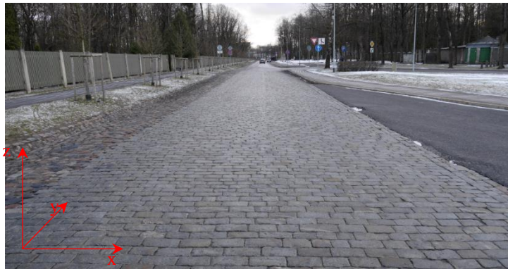
Fig. 1. Cobblestone paving in city made of processed stone. Well maintained
